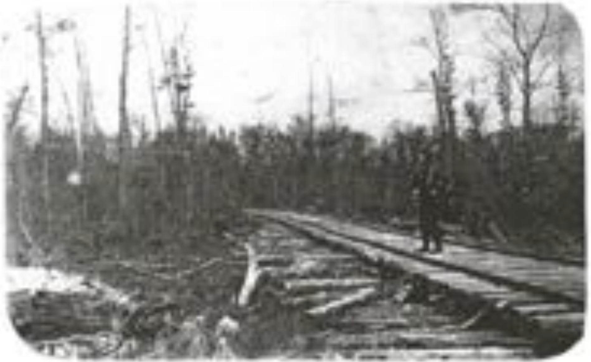
Swamp Poling: akin to corduroy road construction
